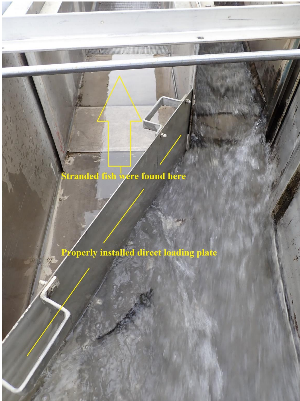
Picture 1: Direct load flume plate properly installed.
